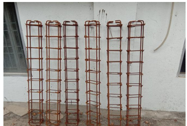
Figure 2 Reinforcement for Beam
